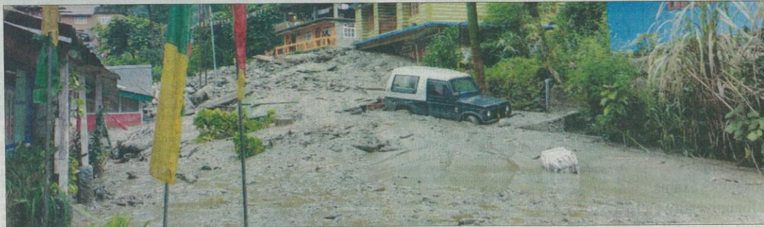
The landslide left behind a trail of devastation at Passingdong village on Saturday night.
