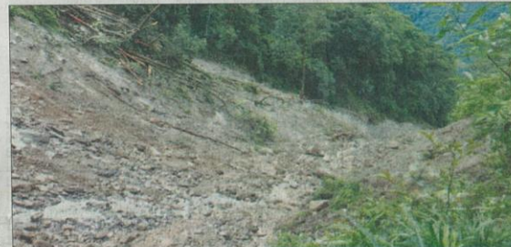
The Passingdong slide had avalanched from Panang area, around one km uphill from the village. The slide is still active and poses threat to settlements below.
