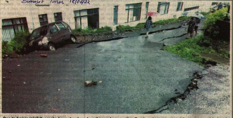
Due to heavy rainfall, cracks have developed on the road connecting Tourism department and Commerce and Industries department. The wall attached to the Tourism department has also been damaged.
